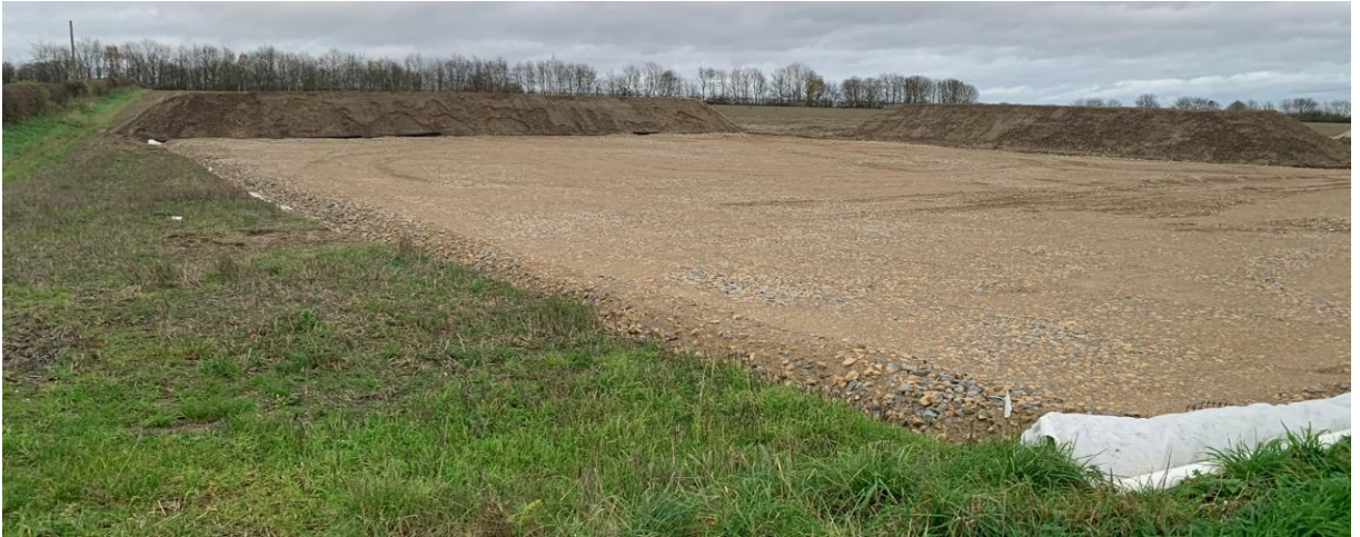
Photo 14: Newly laid Construction Compound (Elsham–Lincoln Pipeline)
